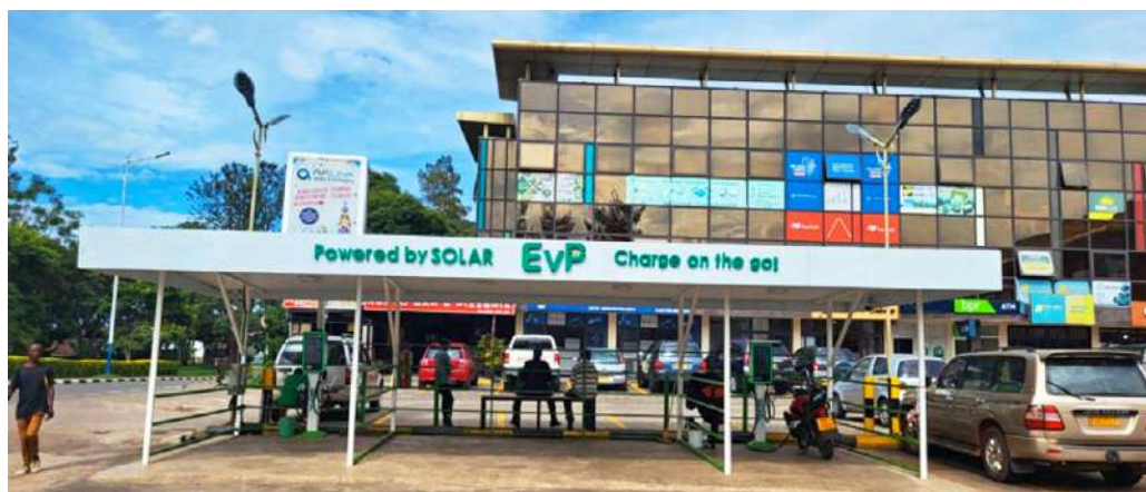
FIGURE 16. Solar powered charging station for electric vehicles in Kigali, Rwanda Source: Moses Ogutu, IAP staff
