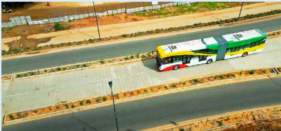
FIGURE 31: Dedicated bus rapid transit lane in Dakar, Senegal Source: Chen, et al. (2023)
